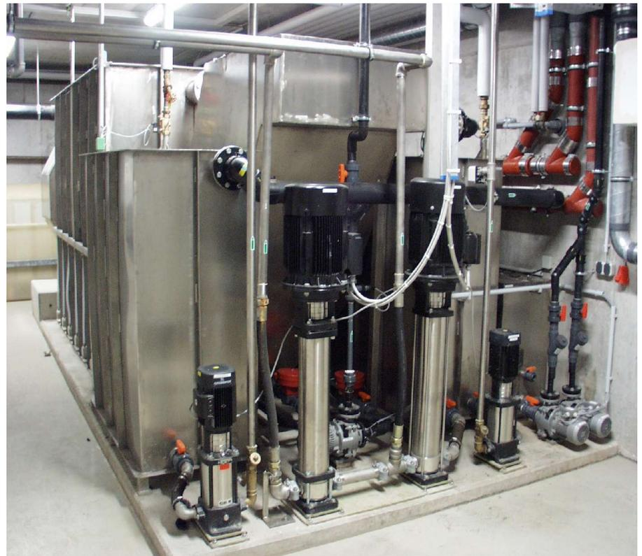
BioClassic System set up above-ground from inside cleaning of bio-waste collection vehicles, with recycling system
